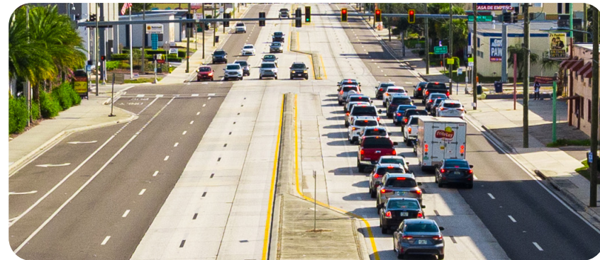
Access Management: Create directional left turn lanes along the corridor to reduce existing conflict points within two-way left-turn lane.
