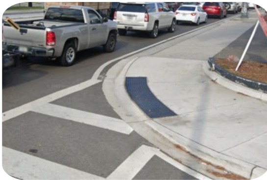
Reduce Curb Radius: Tighten the existing curb radius to slow turning vehicles.
