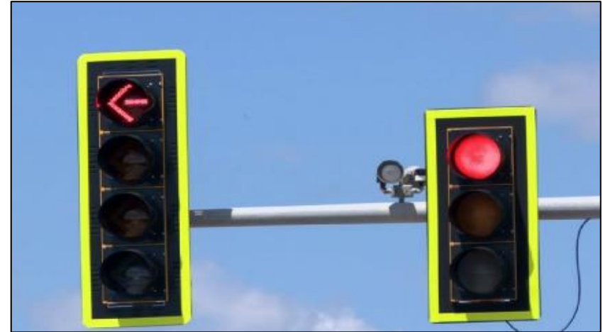
Retroreflective Backplates Suggested to be Considered at E. 19 th Avenue.
