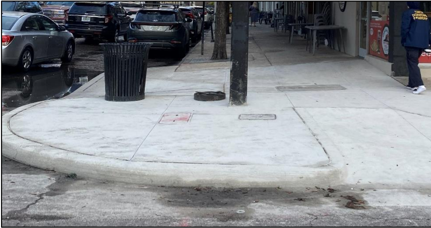
Intersection with Curb Extension Suggested to be Considered at E. 17 th Street.
